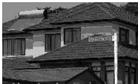
Thermosiphon Flat Plate System
