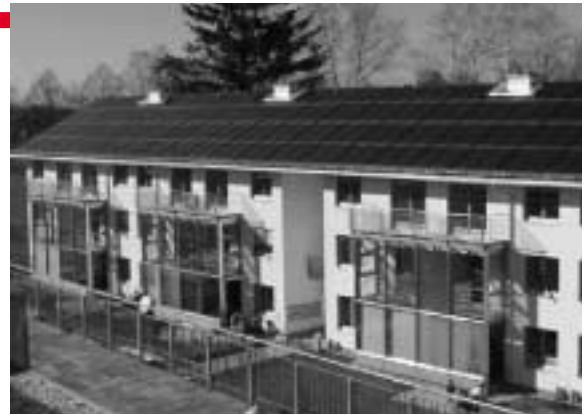
35% of hot water and space heating met by the solar combisystem in this 62-apartment housing estate in Salzburg, Austria.
