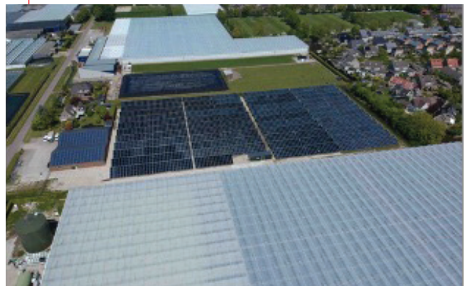
▲ A 6.5 MWth collector field heats a greenhouse in Heerhugowaard, the Netherlands. Photo: G2 Energy
