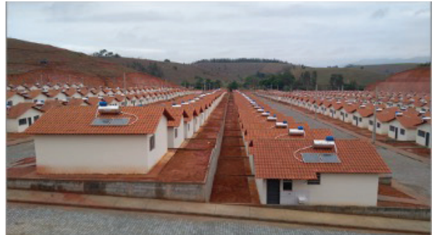
▲ Brazil's Minha Casa, Minha Vida social housing programmes included installing around 400,000 thermosiphon systems. Photo: Tuma
