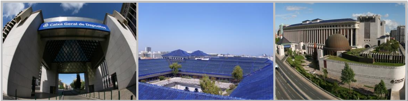
Figure 1. Pictures of the Caixa Geral de Depósitos installation
