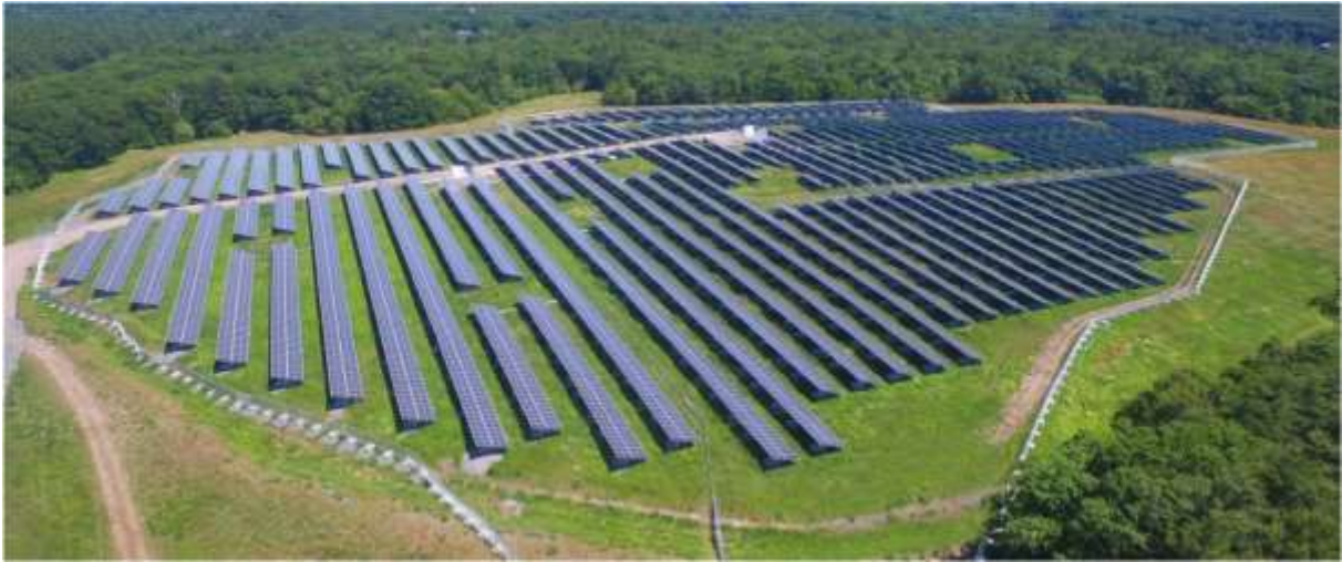
Figure 1: Picture of a 5MW solar development that was built on a 15-acre closed landfill in Beverly, Massachusetts, demonstrating how solar developments can breathe new life to unproductive land. Credit: BlueWave Solar.
