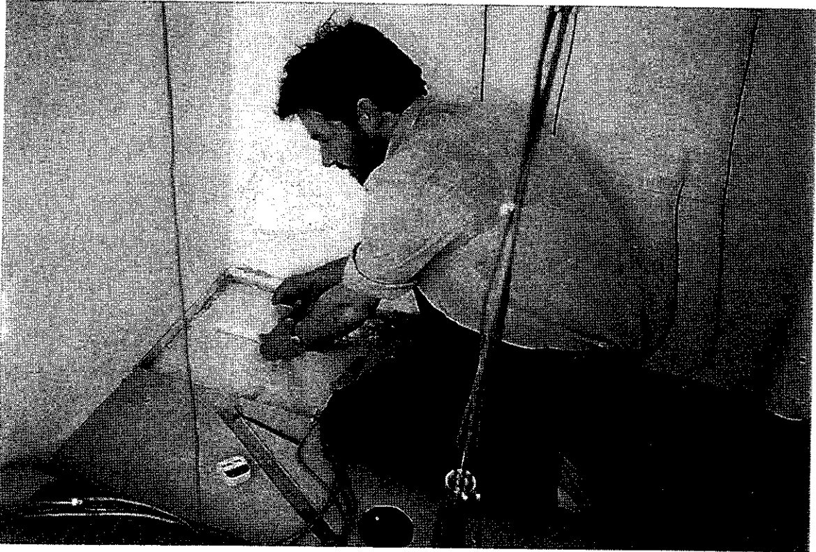
Figure 2.1: Dismantling the test room floor
