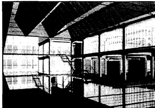
Figure 13.23 Visible photovoltaic panels above the entry hall.
