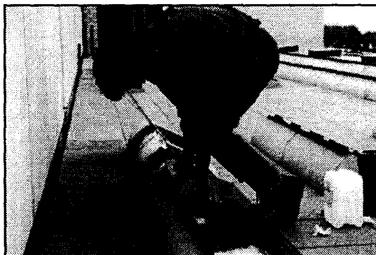
Figure 19.8 Flat roof installation: Glueing of PV modules to concrete block.
