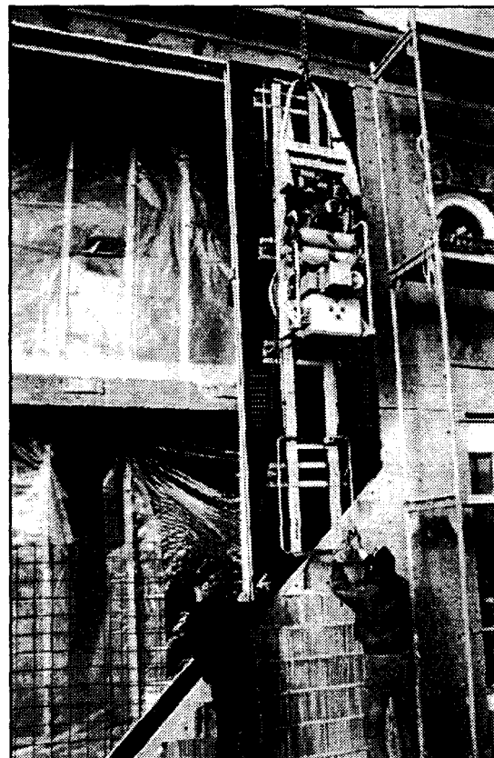
Figure 19.2 Structural glazing: The first facade element is being mounted.
