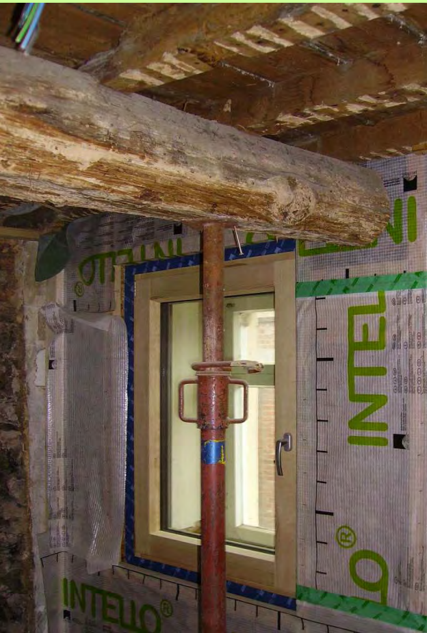
Problem of air tightness on old beam
